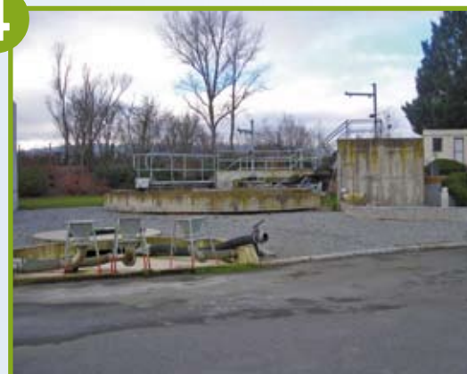
Station d'épuration Etang Bailly
